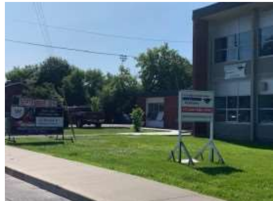
Parking Lot (east side of academy)
